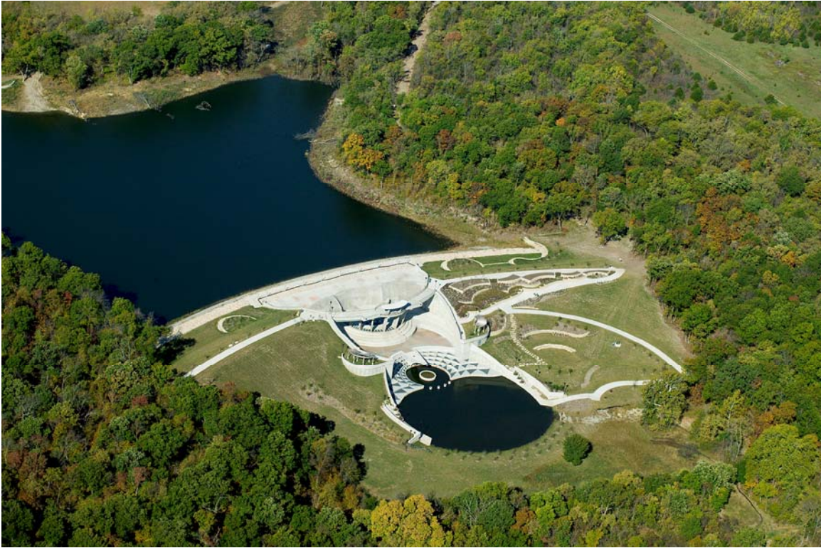
Lake Lenexa Spillway and Dam
